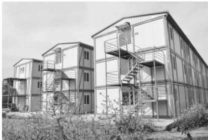
Fig.2 Typical man camp in oil&gas field
